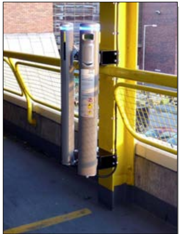
Wall mounted Elektrobay with custom bracket
